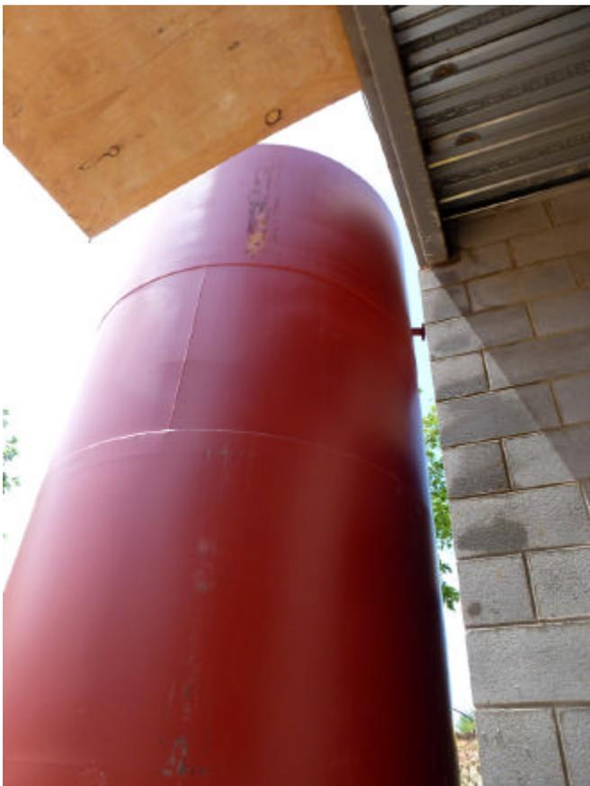
Close up photo of 15,000 gallon water tank. It does not appear to be insulated at this time.
