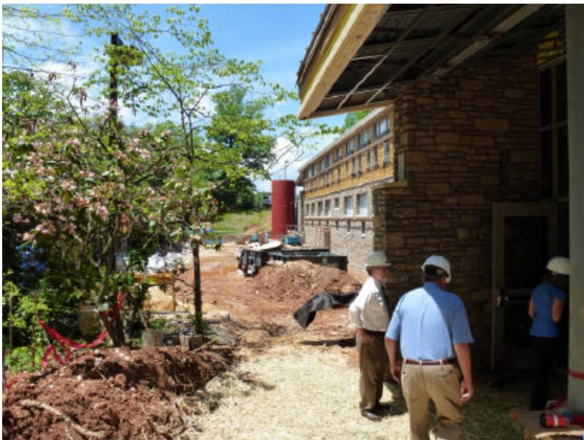
Lower entrance. Far off in the distance is a rust colored 15,000 gallon water storage tank for the solar thermal system.
