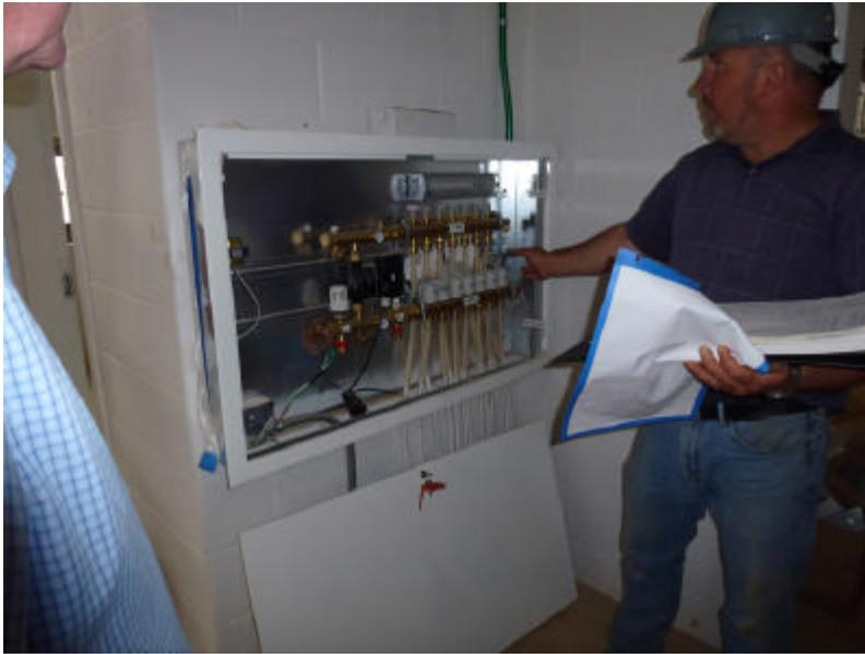
One of the many, many, many control boxes for the flow of heated/cooled water through Pex piping encased in solid concrete in the floors.
