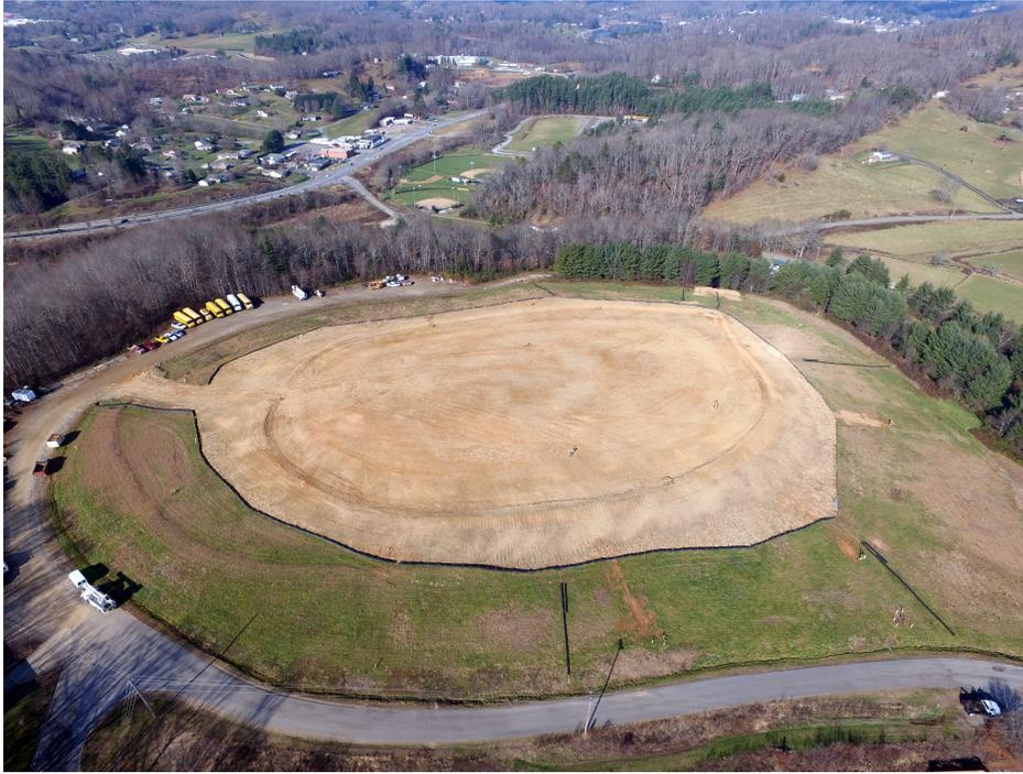
This shows that work seems to be completed smoothing out the dirt on the dome. Plumbing appears to have been added to raise the monitoring well stuff to the new elevation. There appear to be drainage pipes emanating from the dome, and there is a dirt barrier surrounding the new dirt pile. It does not look like a construction zone, as henchman Randy Siske had indicated.
