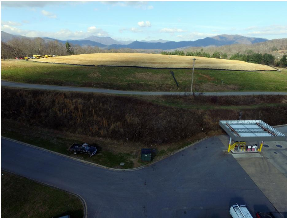
Nearly level with the top of the dome. Notice there is no protective water shedding anything on the top of the dome, just dirt.
